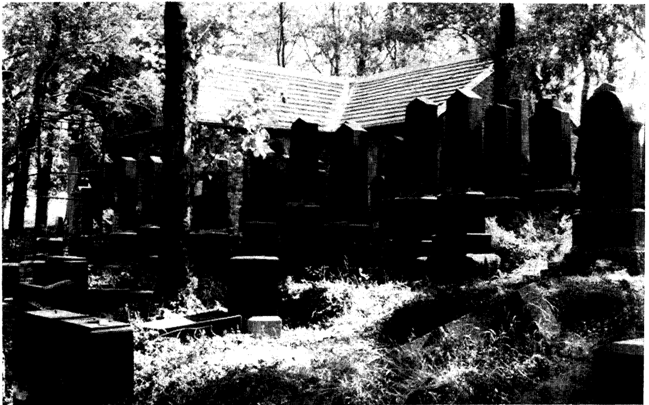
top: Příbram. The cemetery has been cleared of excess vegetation and the walls have been repaired. (Photo: Mojmír Malý, 1992)
