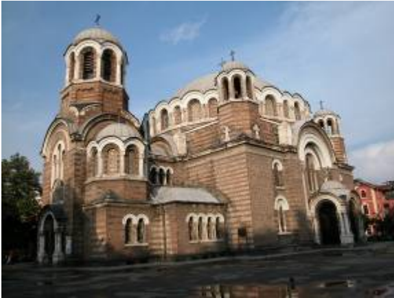
Oblique view showing entranceway/bell tower and vestibule of church and original cube and dome of mosque. Towers and corners, cupolas and arches over lateral entrances, crinolined arches around dome, etc. obscure original clean lines of mosque.
