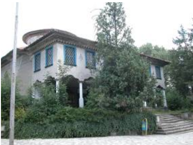
Oblique view of front. Note second story over portico. This space housed the mosque's former medresse .
