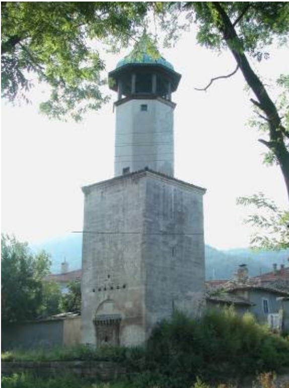
The Clock Tower. The Clock Tower Mosque was located behind and to the right of the tower, just outside the frame of the photo. Note the fountain at the base of the tower. The six holes just above the fountain were sockets for wooden beams that had once supported a wooden eave that protruded out over the fountain.
