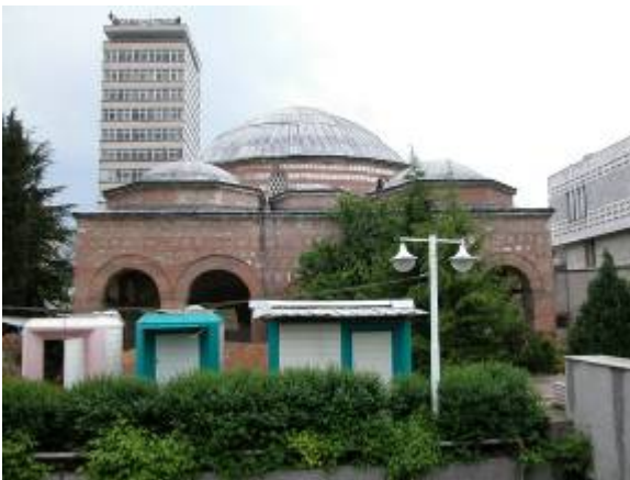
Frontal view of mosque. It is possible that the three domes over the portico are the product of later (possibly 18 th century) renovation. The six-pier, five-arch design of the portico ordinarily would suggest the presence of five domes, one over each arched space.
