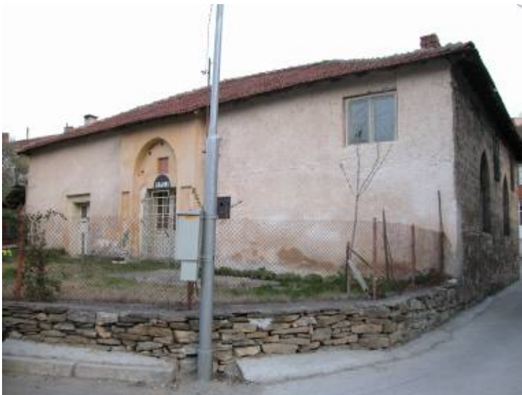
Oblique view of façade and entrance.
