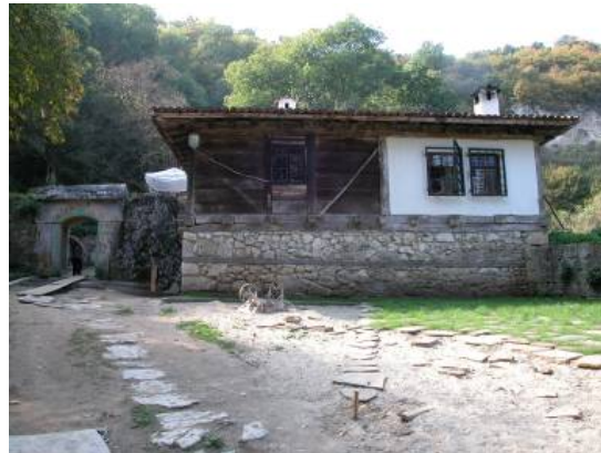
Approach to complex. Gateway at left; rear of imaret/mezdan structure at right.
