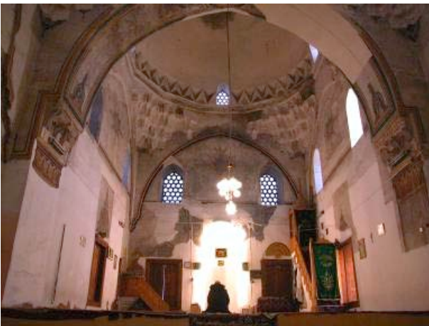
Sanctuary as seen from central vestibule. Note the Turkish-triangle decorations along the drum under the dome and the large muqarnas (a type of corbel, which is a piece of stone jutting out of the wall to support any weight resting on top of it)-decorated pendentives.
