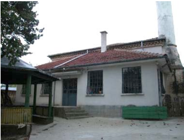
Portico. Şadravan visible at left.
