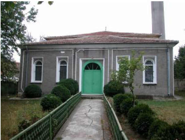
Entrance through walled-in portico.
