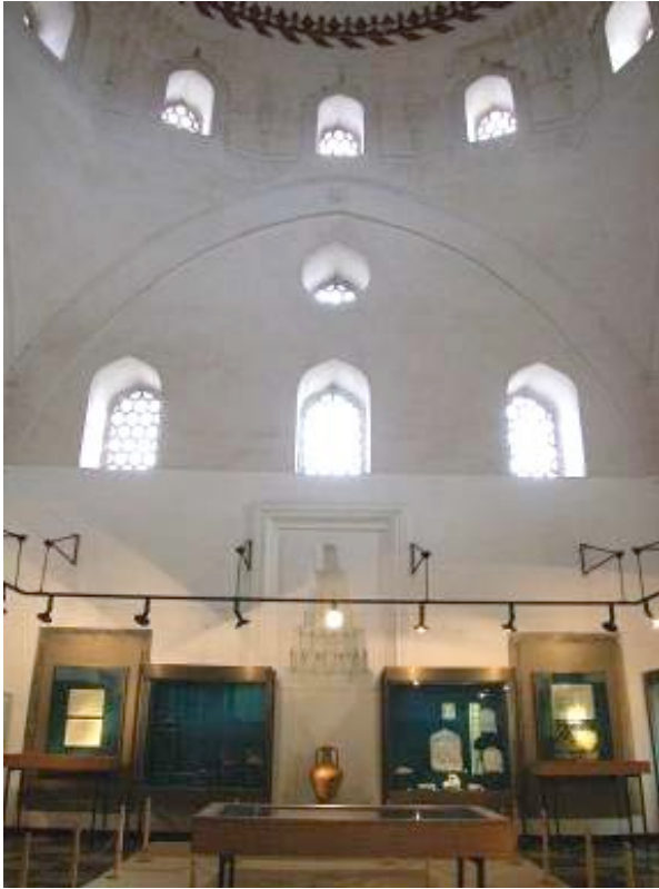
View of qibla showing massive arches and pendentives that support the walls of the sanctuary. The soaring interior is well illuminated by windows penetrating three of the walls and the twelve facets of the drum of the dome.
