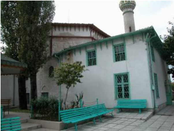
Oblique view from within the courtyard of the mosque showing bricked-in portico, cut stone wall and straightforward octagonal drum housing the dome. A part of the modern eave of the şadravan is visible at the left.
