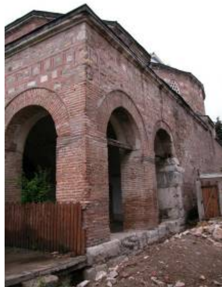
Close-up of piers. Note that the piers are of brick. Also note the high-quality of the cloisonné work and that the portico and sanctuary are of a single piece. Signs of excavation work are visible in the foreground.
