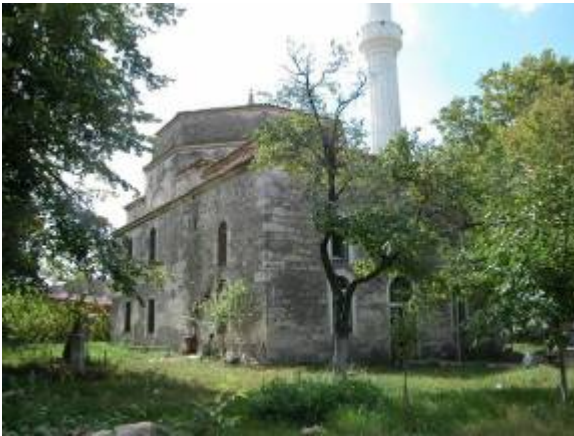
Oblique view facing front of mosque.
