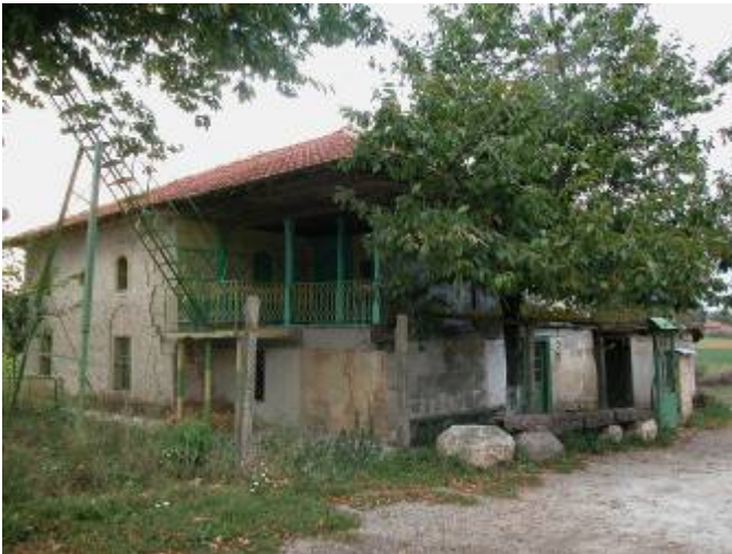
Exterior. Note shifting of stone blocks near the front of the left lateral wall of the sanctuary. Also note the inclined fireman's ladder-like stairway to the minaret. Minarets of many urban and rural mosques in Bulgaria were ordered torn down or were forcibly razed during two decades of officially directed and often popularly supported anti-Turkish and anti-Muslim campaigns during the 1970s and 1980s.
