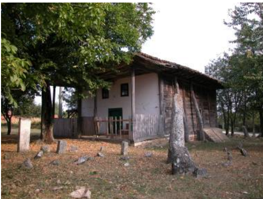
Oblique view to front of mosque from right. Remains of cemetery in foreground.
