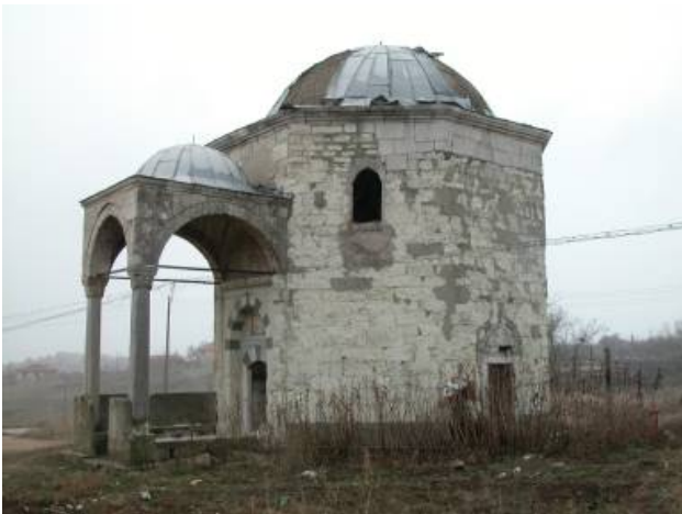
Lateral view. Note alternate placement of upper and lower windows.
