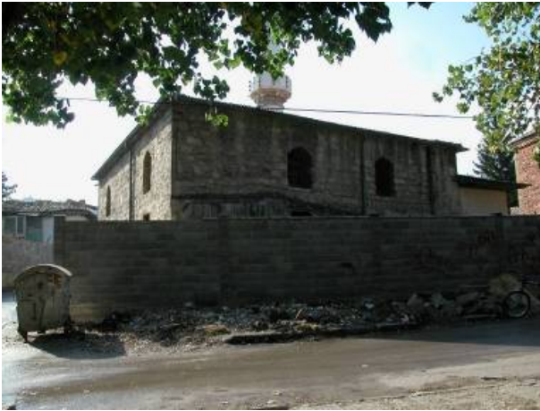
Lateral view from street. Note qibla wall at left and enclosed portico at right.
