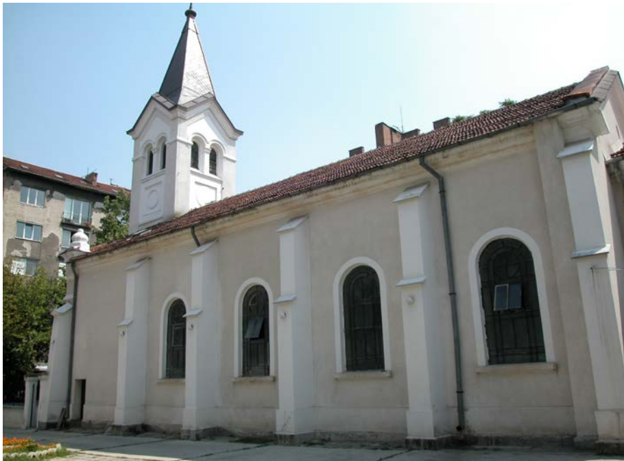
Side view with tower.
