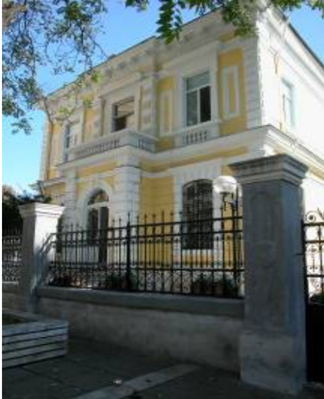
Pastor's house, from street.
