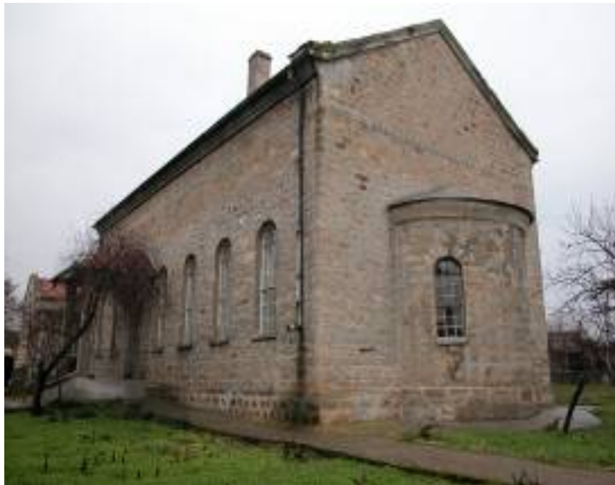
Rear (altar end) of church and lateral wall from street side of courtyard. Note apse (with signs of extensive repair) and (at left) main entrance to the church through lateral wall. Pastor's house is visible at the extreme left.
