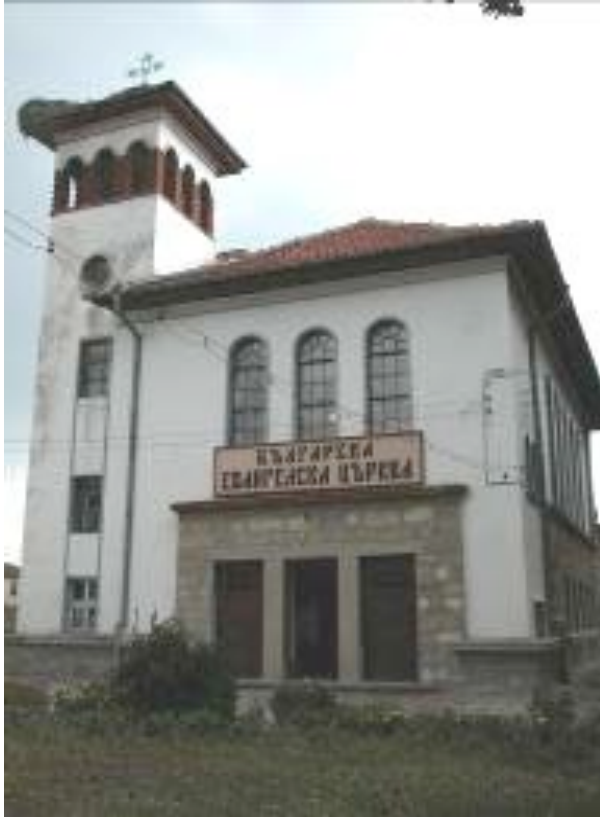
Frontal view. Note cut-stone portal.
