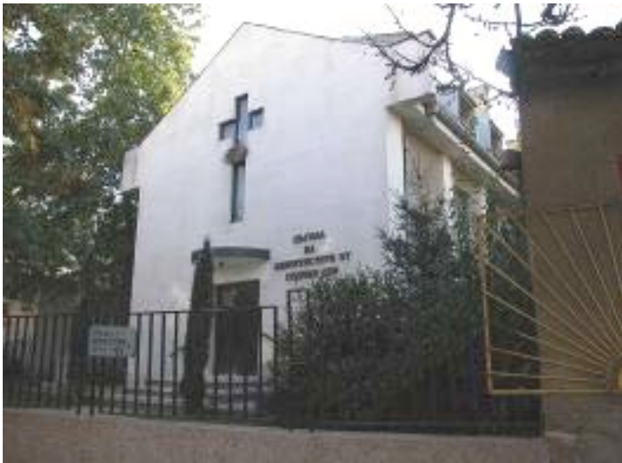
Oblique view of façade and right wall of church from sidewalk.
