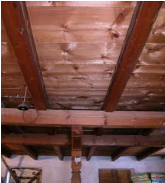
View of wood floor construction and beam supports. Taken from ground floor looking upward.
