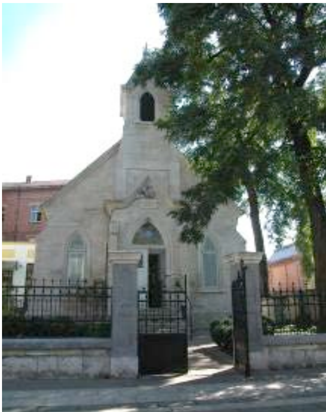
Façade from street.
