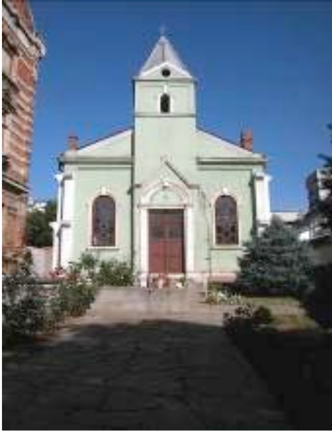
Façade, from courtyard.
