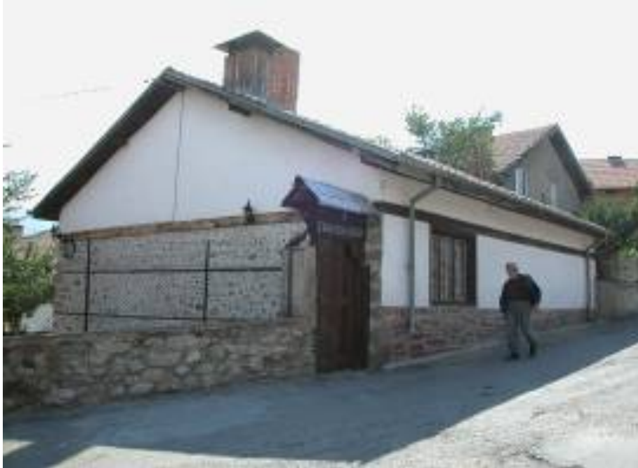
Oblique view from front street. Note traditional stonework with exposed beams of wood frame, traditional stone wall, and courtyard entrance portal.
