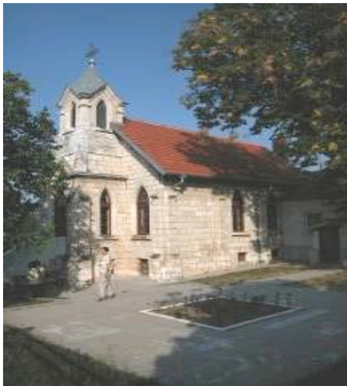
Diagonal view from courtyard. Note pastor's house abutting on church (partially visible in shadow at right).
