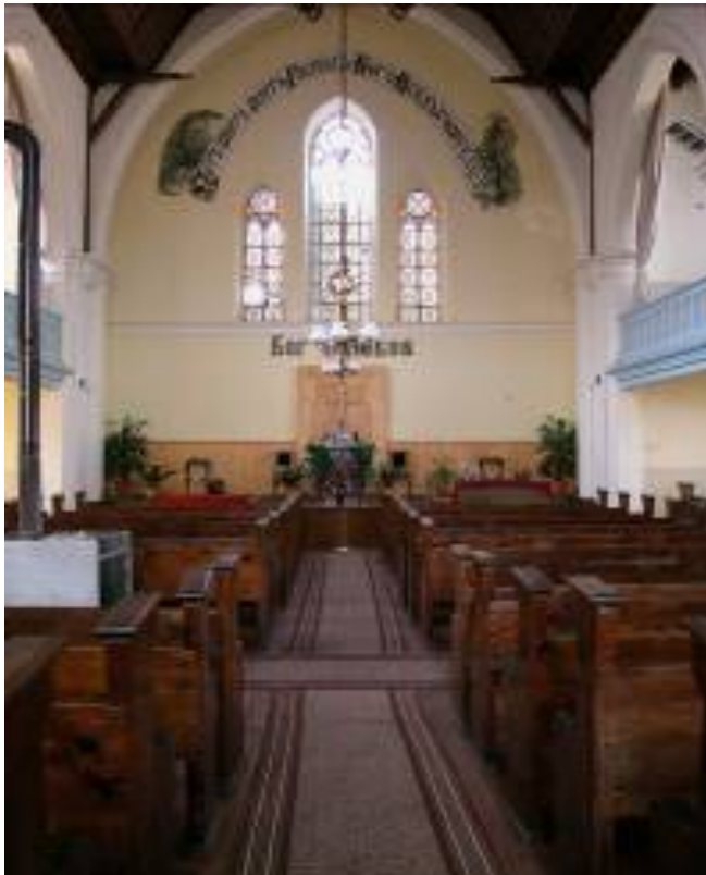
Interior, toward altar from rear of church. Note the neo-Gothic piers and spring of arches.
