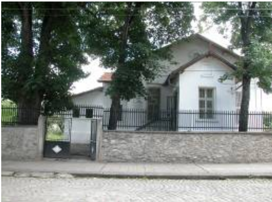
View from the street. Note that a pitched attic had been about two meters higher in the original structure. The second story and the bell tower (originally at the left of the church) were destroyed in a fire a century ago.
