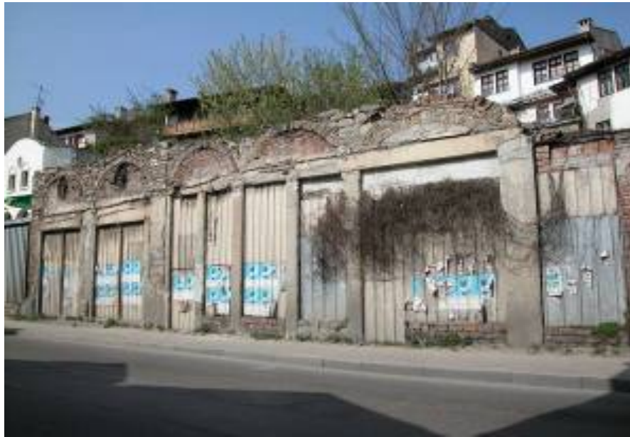
Remains of façade from right.
