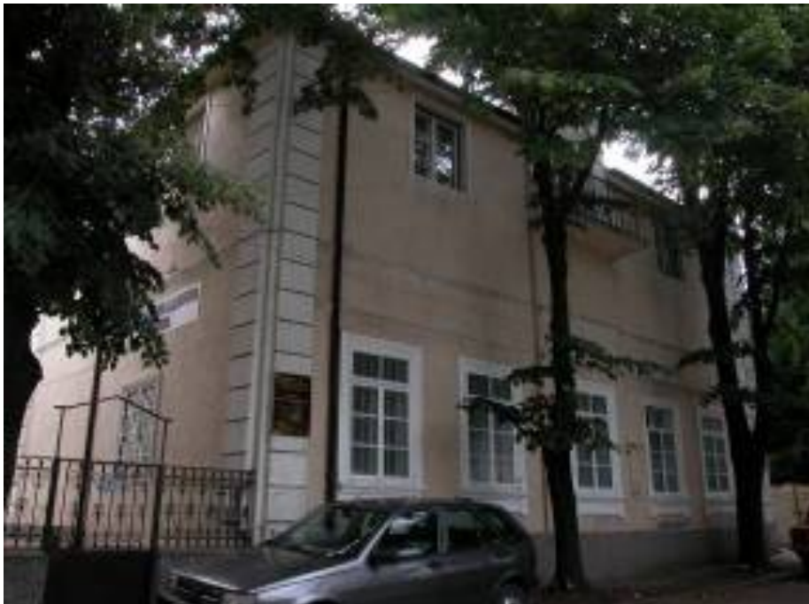
Building as seen from the street. Entrance is at the far left.
