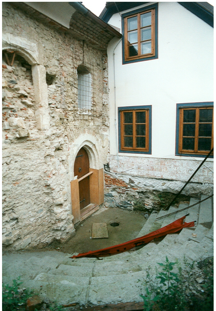
Figures 35, 36. Maribor. Synagogue. Top: Detail of north façade. Bottom: Detail of north façade with new entrance stairs and door.
