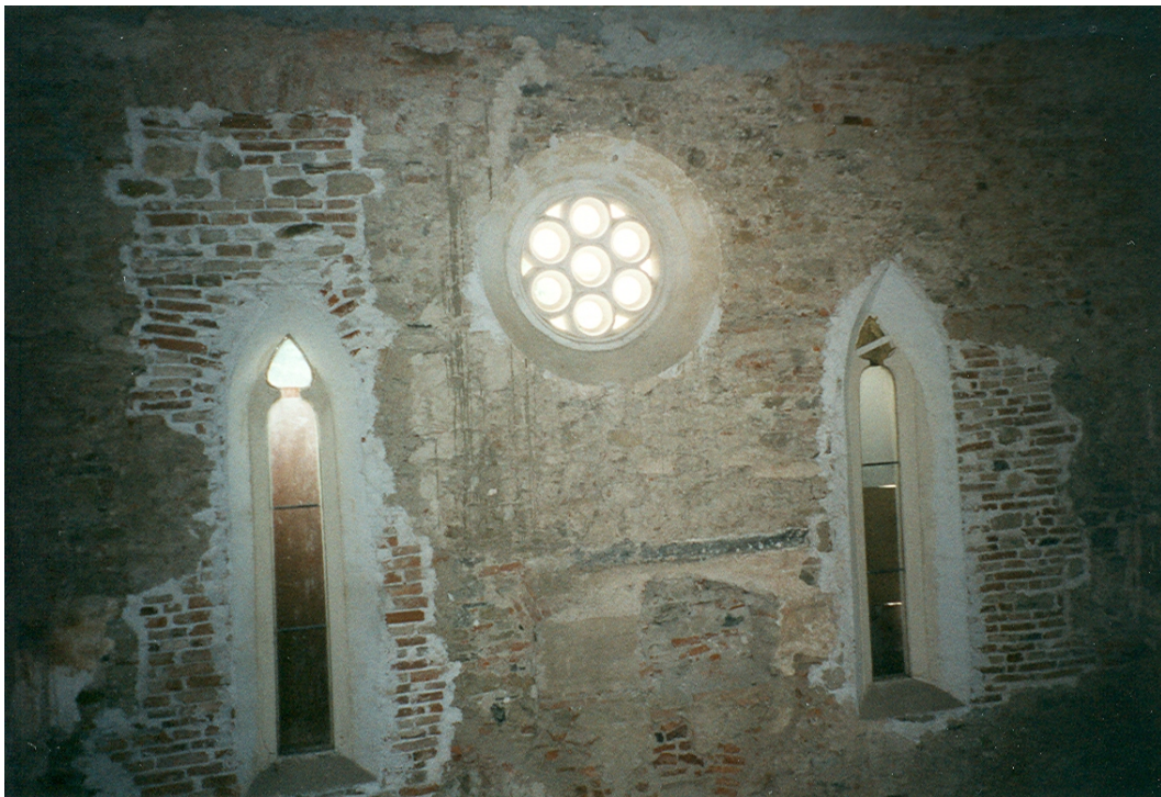
Figures 37, 38. Maribor. Synagogue. Top: Interior after creation of “women’s gallery,” a modern invention which must now be removed. Bottom: Main hall, view of east wall with rebuilt lancet windows and oculus above presumed location of Ark.
